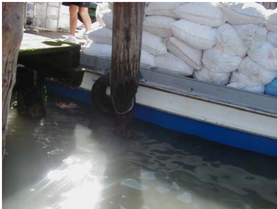
Figure 18: Rotting Dock
