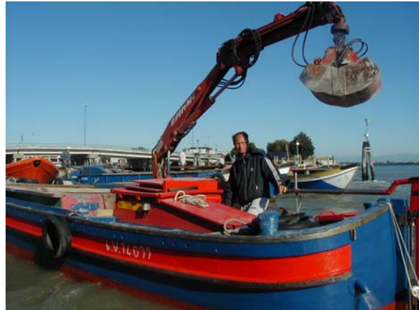
Figure 8: Construction Boat with Crane
