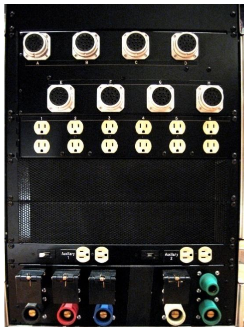
Figure 2 - Rear of a typical dimmer rack.
