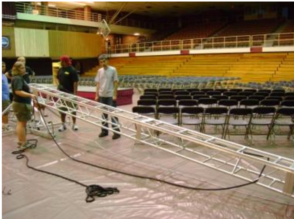
Figure 15: The rope is threaded through the tower so it can be pulled up
