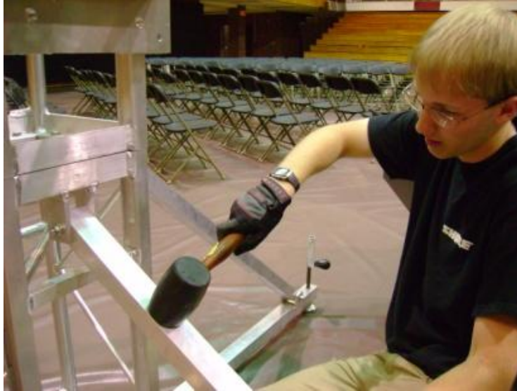
Figure 18: Using the rubber mallet to fit the outrigger into place
