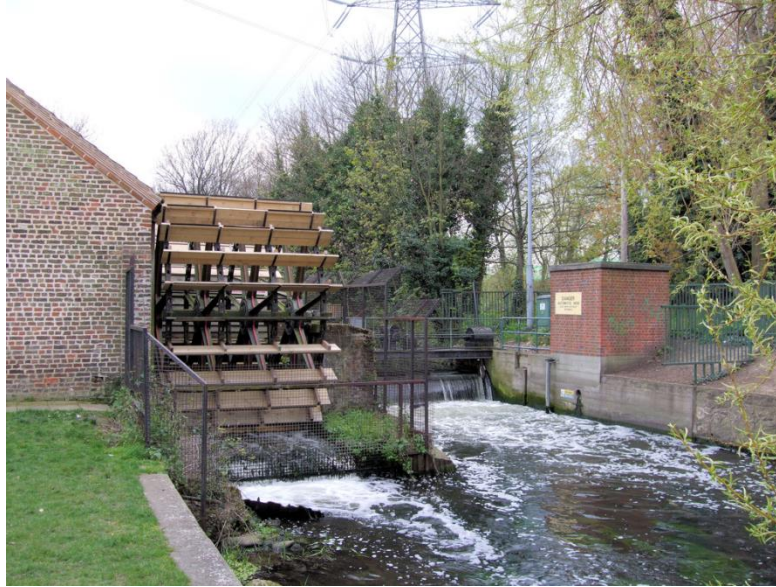
Figure 15. Merton Abbey Mills water wheel Source: (Linwood, 2008)
