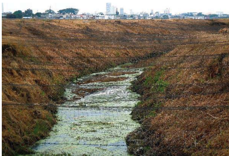
Figure 10: Net system at Guayaquil Airport
