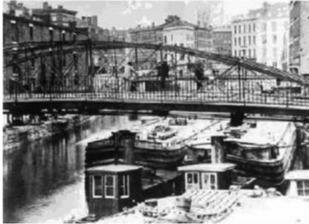
Figure 4: Whipple Truss Bridge circa 1870 (Fonzi, 2008)
