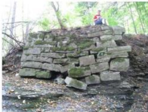
Figure 9: Existing stone abutment
