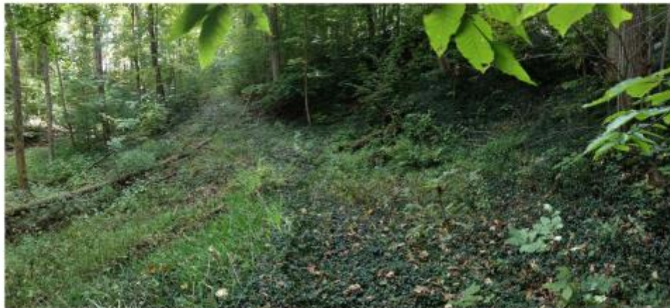
Figure 5: A portion of the proposed ravine trail that experiences frequent drainage issues.
