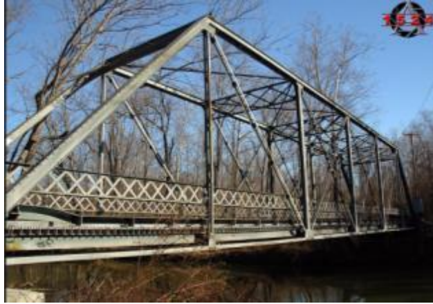
Figure 5: Pratt Truss Bridge http://www.flickr.com/photos/sparks1524/2212838461/
