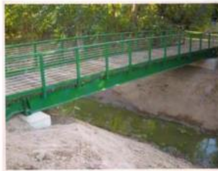
Figure 15: Flatcar pedestrian bridge
