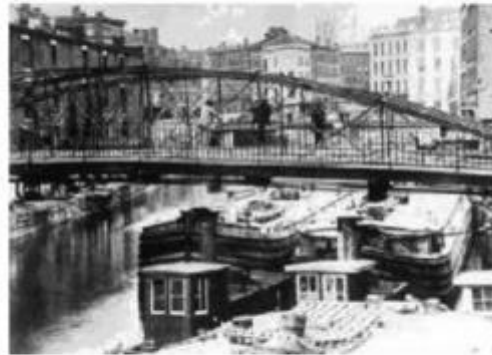
Figure 7: Whipple Truss Bridge circa 1870
