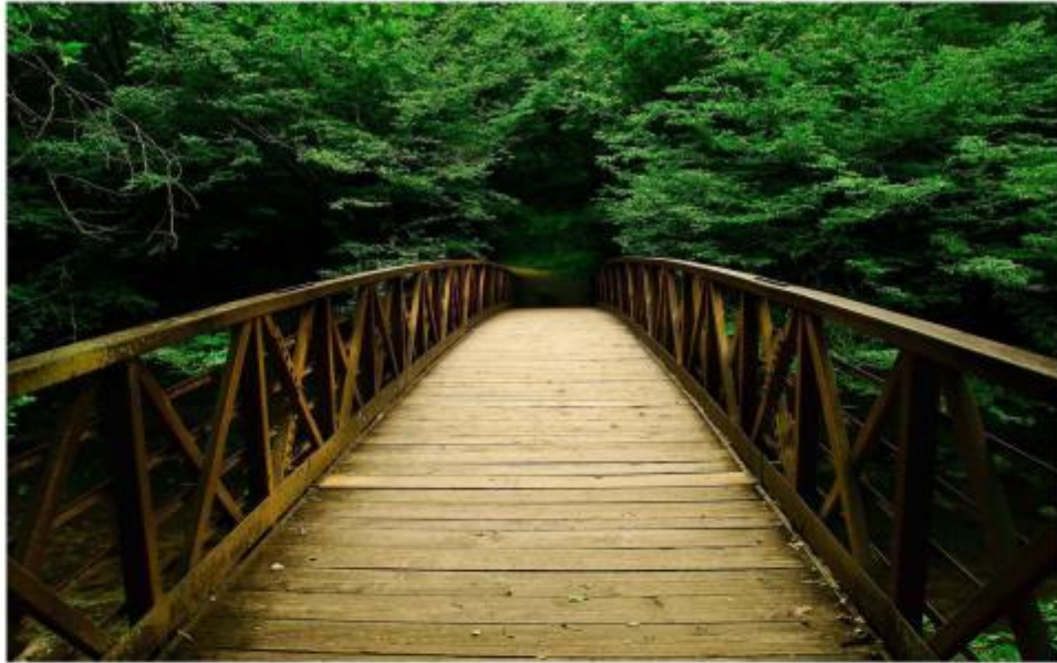
Figure 12: Example of a typical wooden pedestrian bridge
