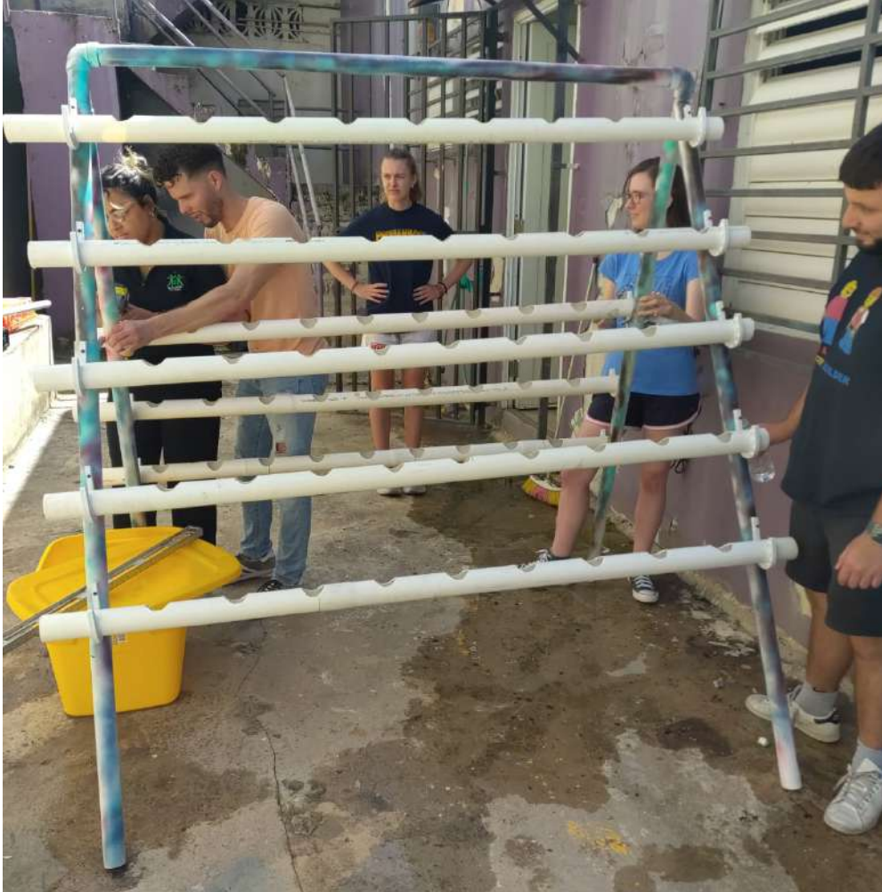
Figure 29: The team working with Glory and Anthony G. Calzada Rivera to assemble the PVC A-frame. Screws were drilled into PVC pieces to attach J-hooks and strengthen the frame.
