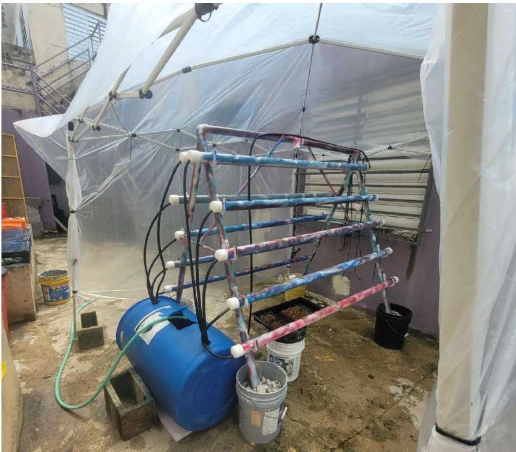
Figure 20: Completed hydroponic garden system, featuring PVC A-frame structure, plastic roofing, rubber tubing, 55-gallon tank, and cement bucket stabilizers.
