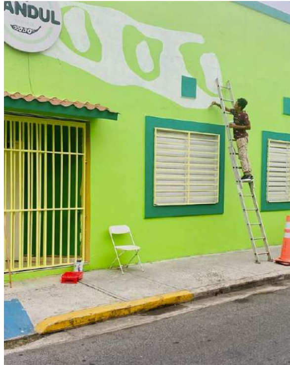
Figure 6: Community members gather to repaint the El Gandul Community Center. March 25, 2023.
