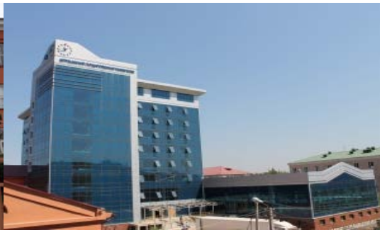
Figure 2.d. The new building at ASU.
