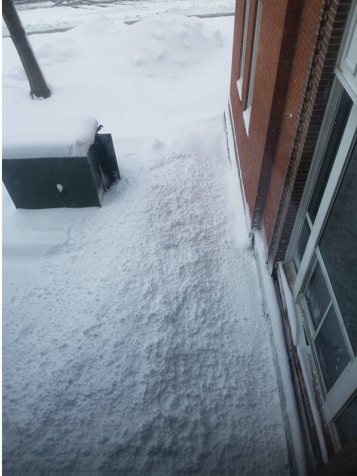
Figure 5: Prospective Snow Damage
