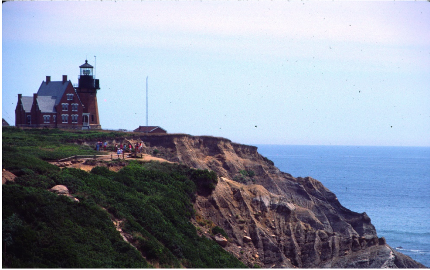
Figure 2-5 The Southeast Lighthouse prior to move. Note the people standing on the bluffs.
