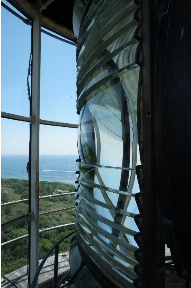
Figure 2-9 A first order Fresnel lens inside the Southeast Lighthouse.
