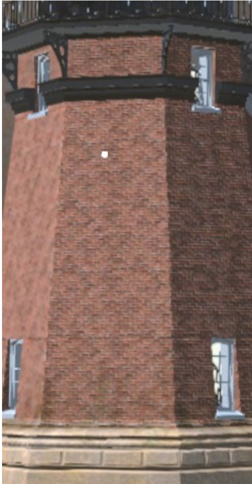
Figure 5-7 A brick surface completed.
