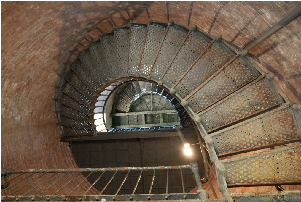
Figure 2-8 Inside the tower looking up through the cast iron spiral staircase.
