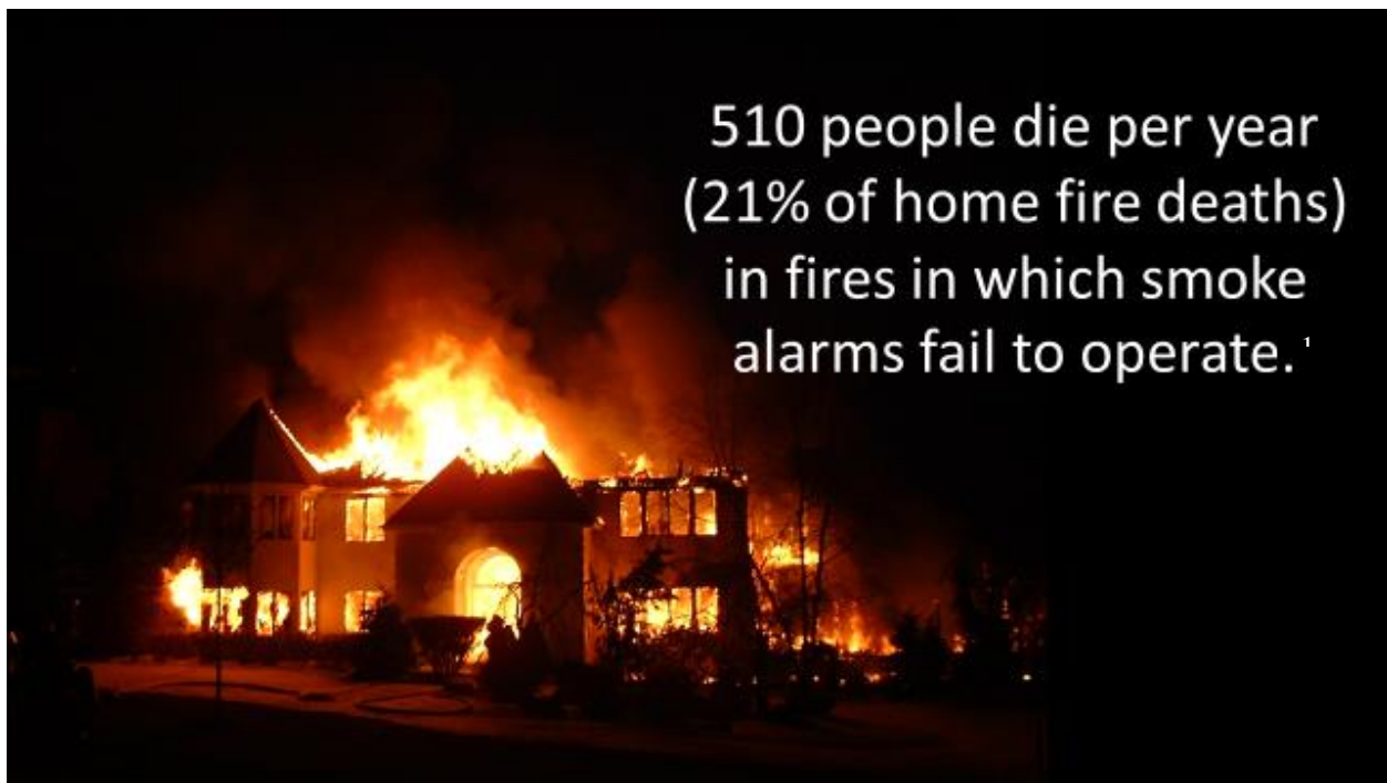
Figure 1: Home Structure Fire (Ahrens, 2015b) 1
