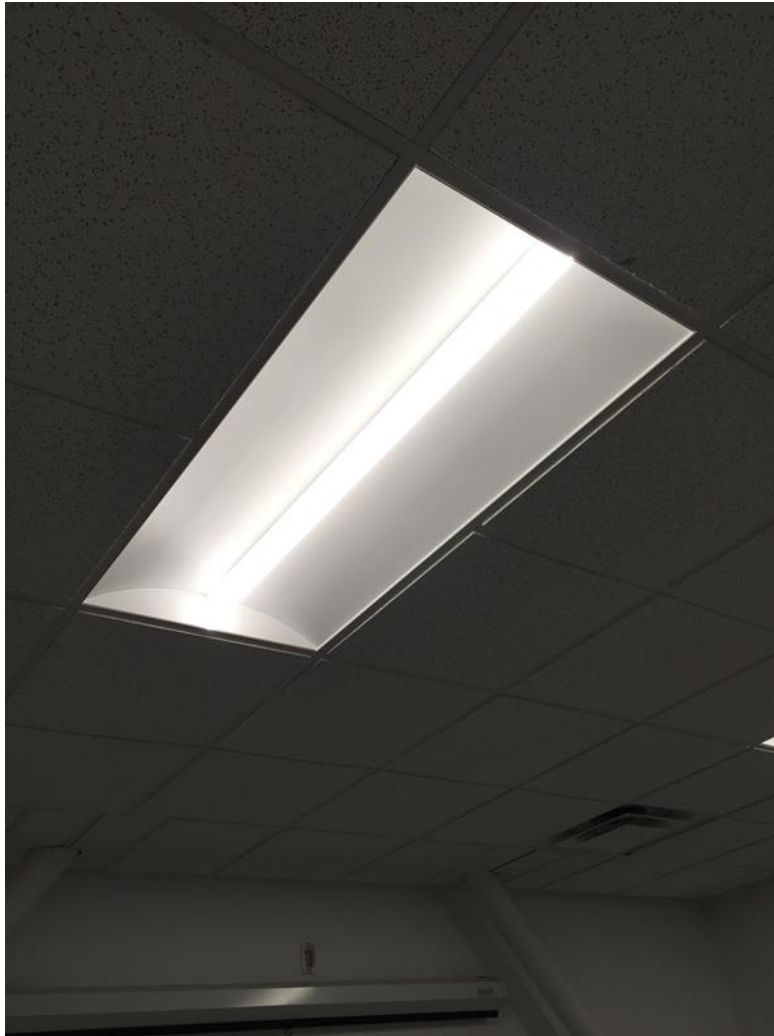
Figure 23: LED fixture replacement
