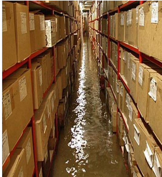
Figure 1: Water Damage at the New Mexico Museum of Indian Arts and Culture in Santa Fe, New Mexico (Heritage Preservation, 2005)
