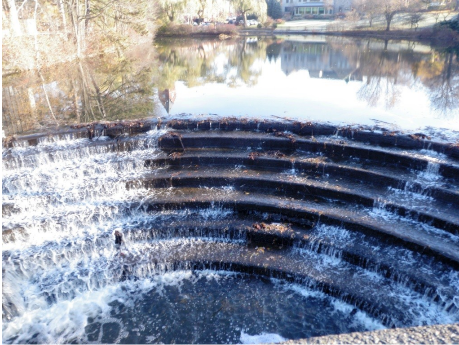
Figure 39: The Center Falls Dam, Winchester MA
