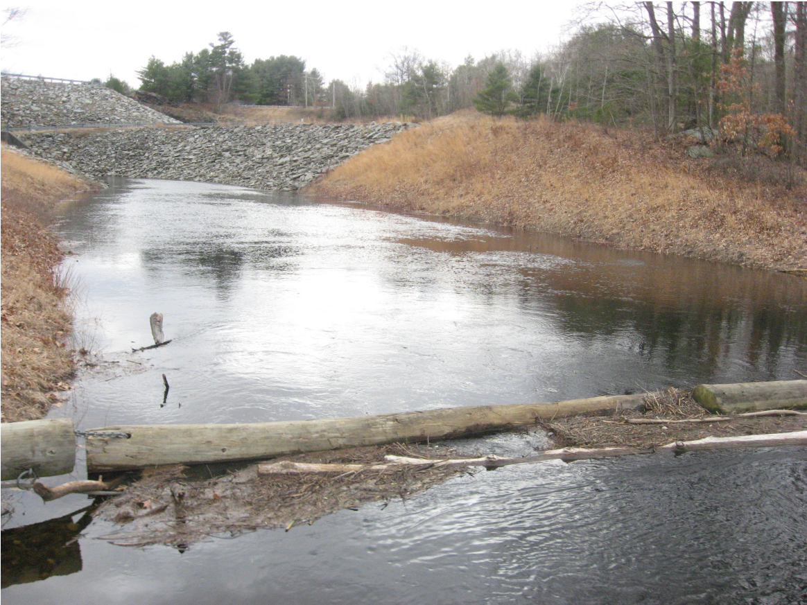
Figure 9: Hodges Village Dam: French River(M8)
