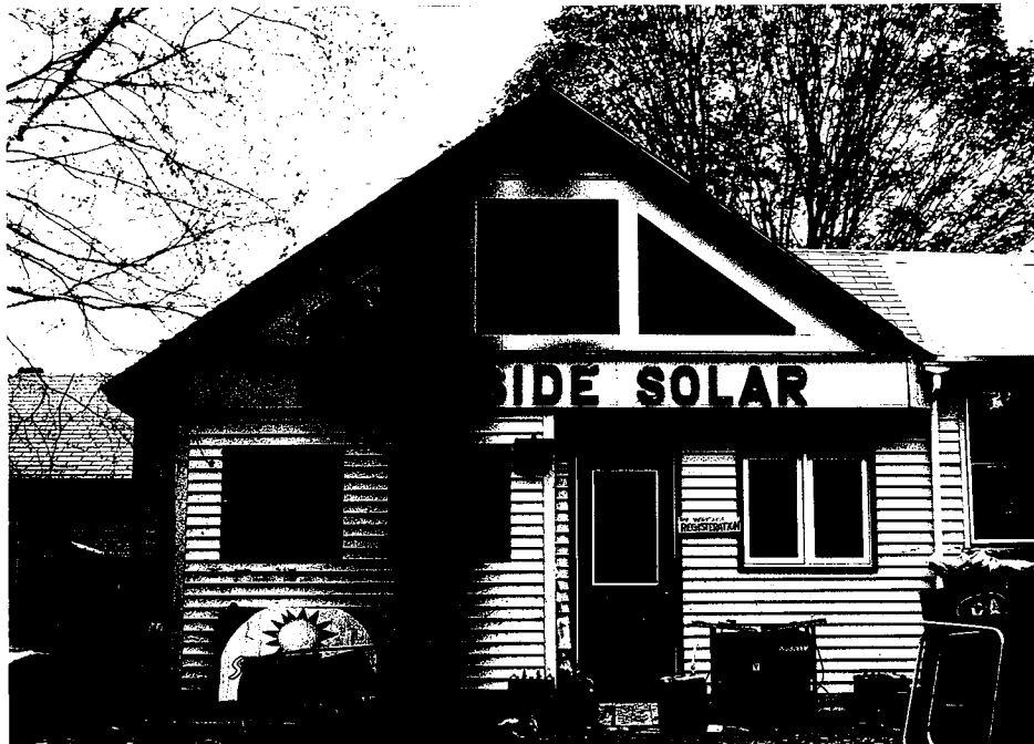
Sunnyside Solar Located in Brattleboro Vermont Pictures taken during workshop in May 1992
