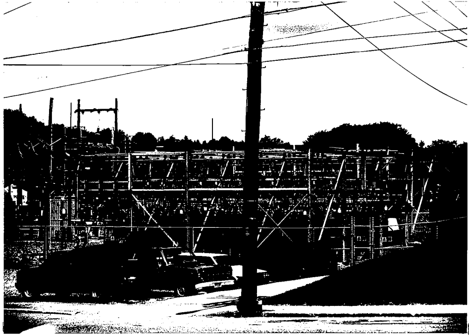
Substation For The Gardner Homes
