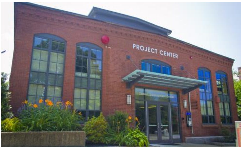
Figure 2: Current Facade of WPI's Project Center
