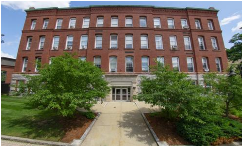
Figure 1: Current Facade of Stratton Hall
