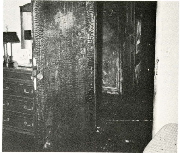
Chicago Fire Department, Chicago, Illinois
