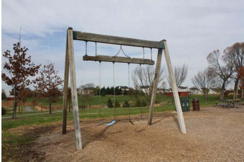
Figure 42: Worn Out Surfacing Around Swings
