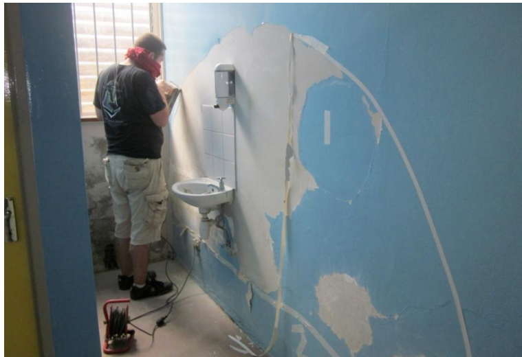
FIGURE 13. SANDING THE WALLS
