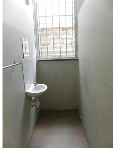
VIEW OF WASH BASIN NEXT TO GENTLEMAN'S STALL
