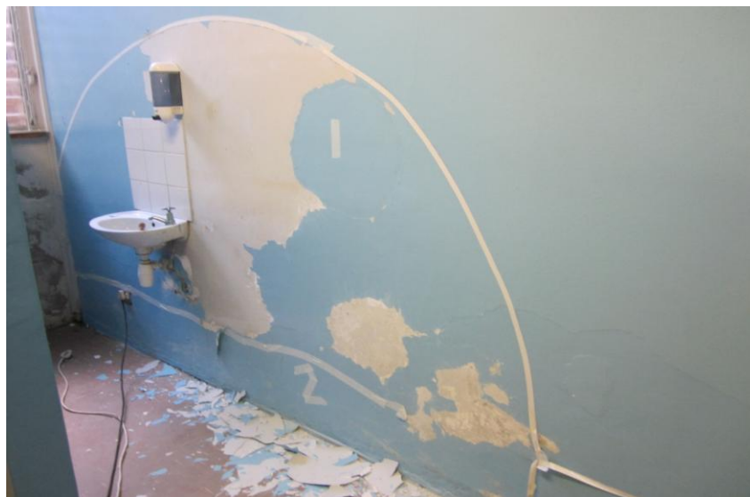
FIGURE 12. STRIPPING THE WALLS
