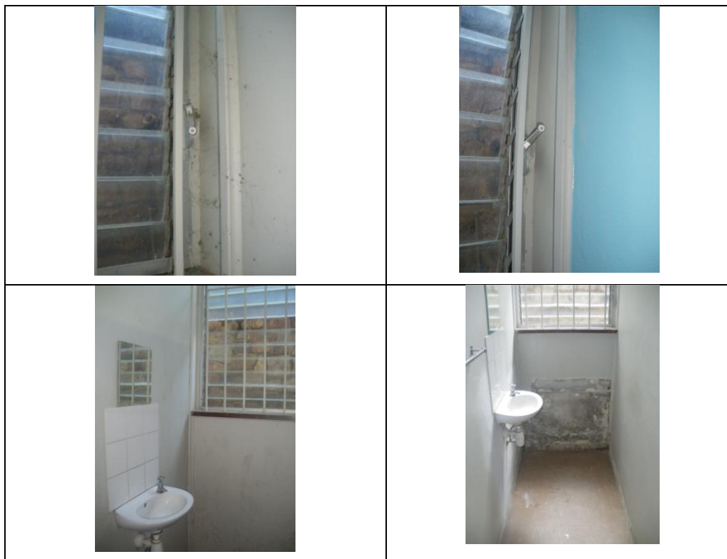
FIGURE 8. CLEANING AND DISINFECTING THE WALLS
