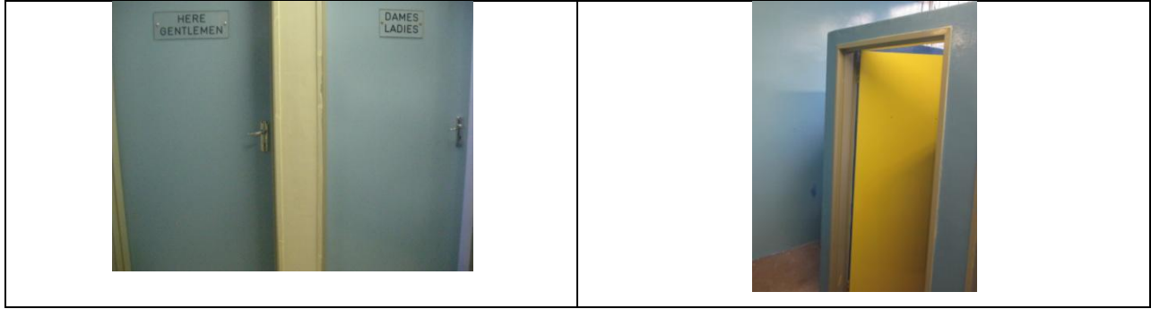
FIGURE 17. VIEW OF STALL DOORS
