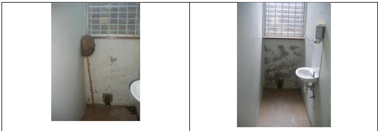
FIGURE 9. SANDING THE WALLS
