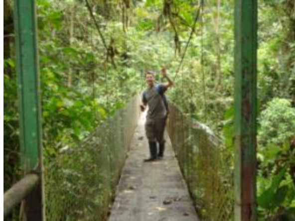
Figure 16 - Existing Bridge at La Marta
