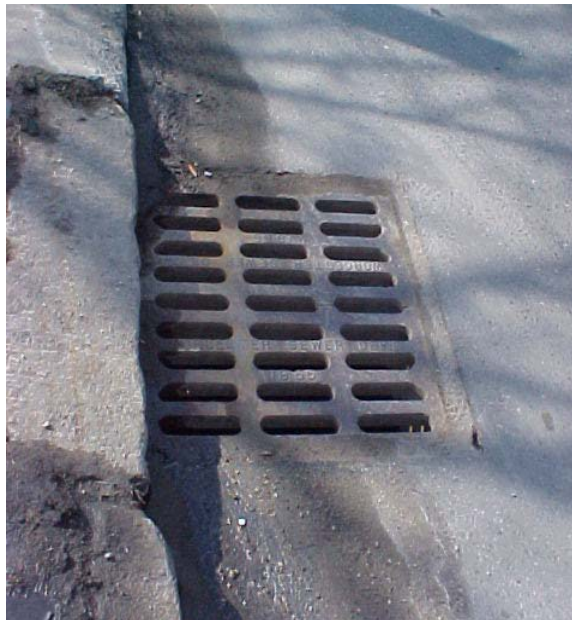
Figure 20: Example of Roadside Drainage
