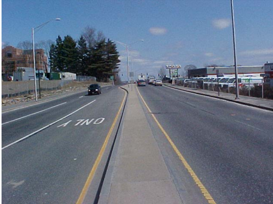
Figure 8: Raised Curb Median
