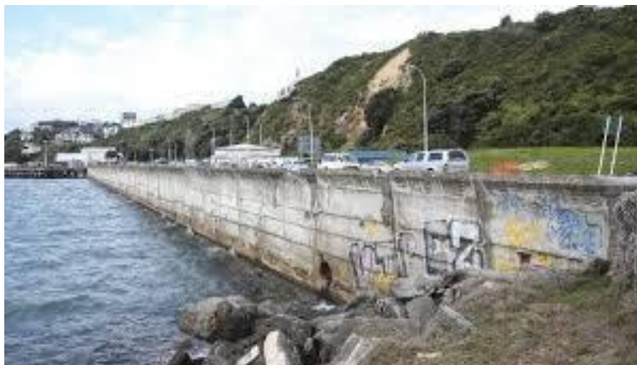
Figure 4. A seawall in Wellington, New Zealand (Devlin, 2018)
