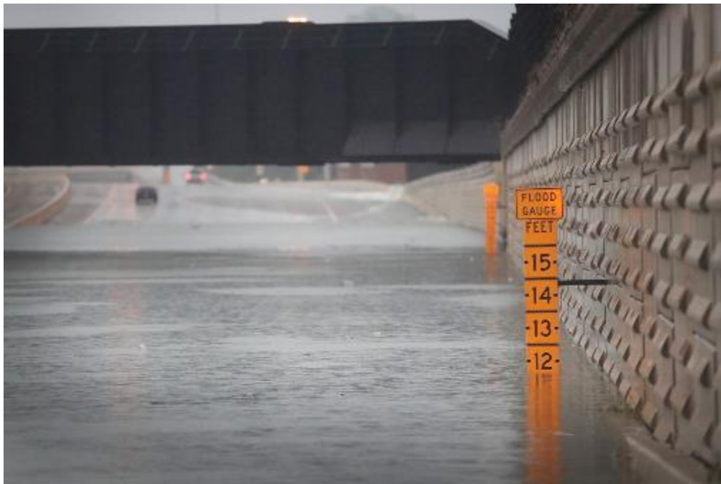
Figure 37. A flood gauge in Houston, TX (Olson, 2017)
