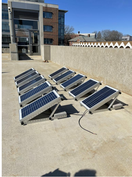
Figure 20: Solar panel set-up on top of the East Hall garage - panels are set up in two rows of five and are weighed down by cement blocks.
