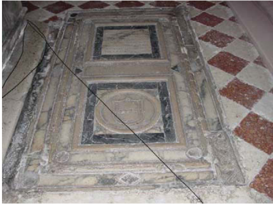
Figure 29: This artifact found in the San Giobbe contained a high percentage of surface cracks
