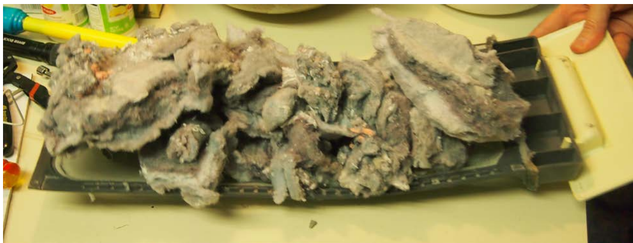
Figure C- 7: Lint Screen and Compacted Lint Removed from Screen Area
