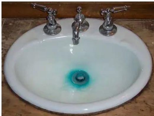
Figure 2. Sink Stained from Copper in Water (Mr. Plumber, n.d.)
