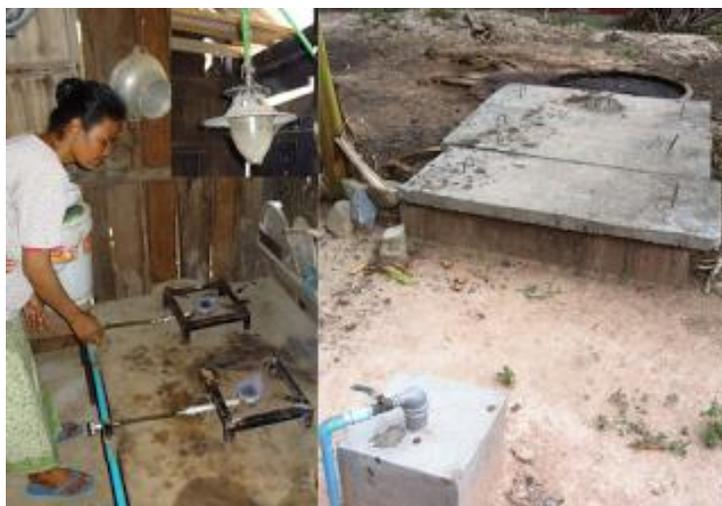
*Figure 11: Biodigester to cooking stove process (Tahezadeh, 2012).*
