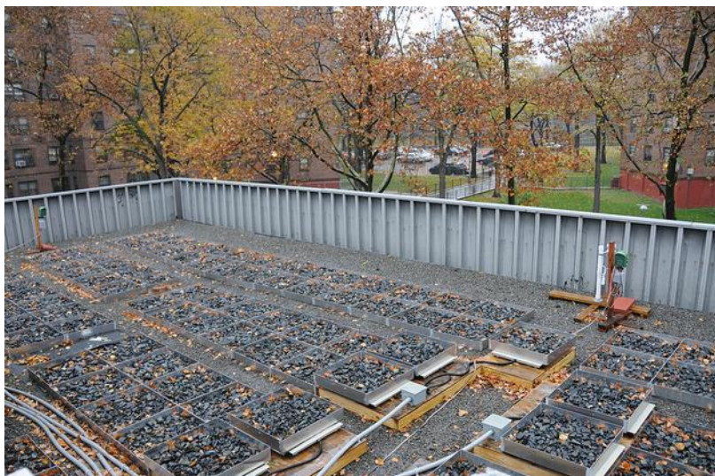
Figure 5: Blue Roof (NYC Environmental Protection, 2012)
