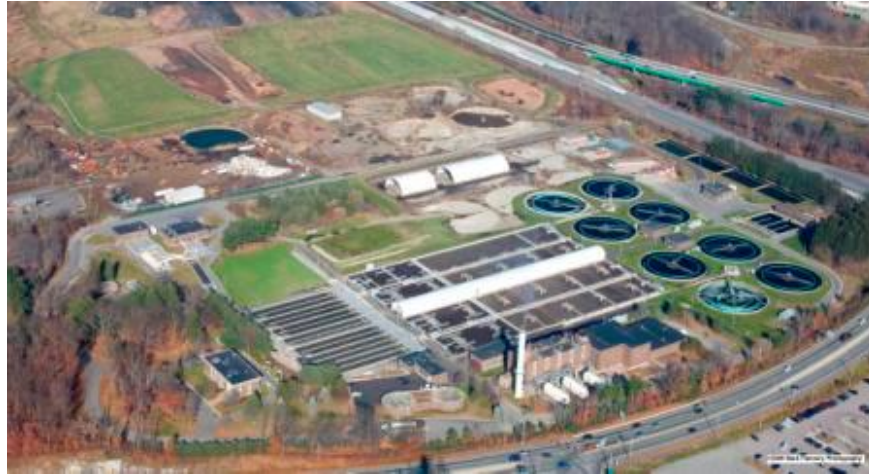
Figure 13: Photograph of Upper Blackstone Wastewater Treatment Facility (UBWWTF) (UBWPAD, 2012)
