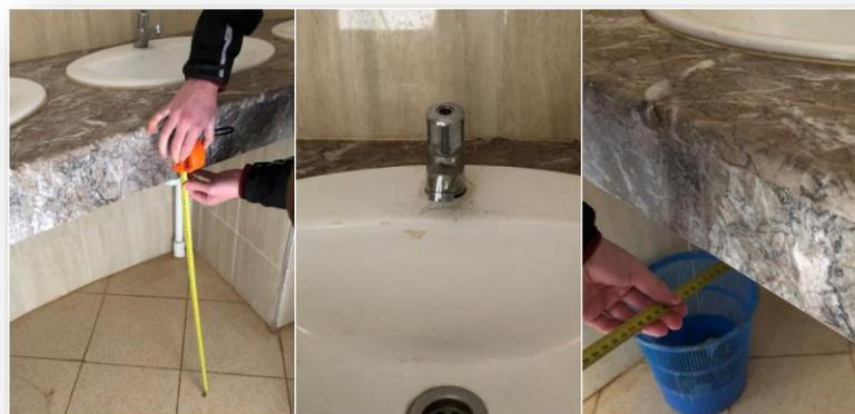
Figure 15: Accessible sink height, operable faucet and sink clearance. January 22, 2020.
