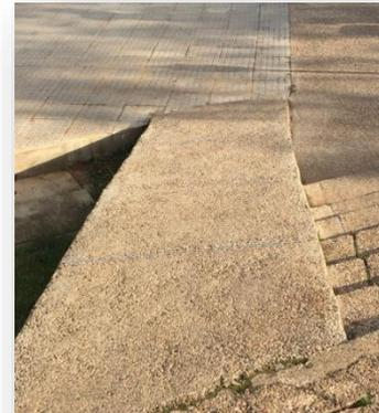
Figure 10: Ramp in front of the library at the FMP-Rabat with slope 1:5. January 16, 2020.
