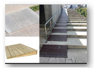
Figure 18 On the left examples of portable wood and metal ramps, and on the right visual image of how the implementation of the ramps can look like. Adapted from "Metal and wood ramp for supporting disabled people wheelchair" by Chuankul (2020).
