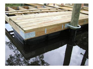
Figure 33: Example of a floating dock that is held in place by stationary posts (Dock Builders Supply™, 2013)
