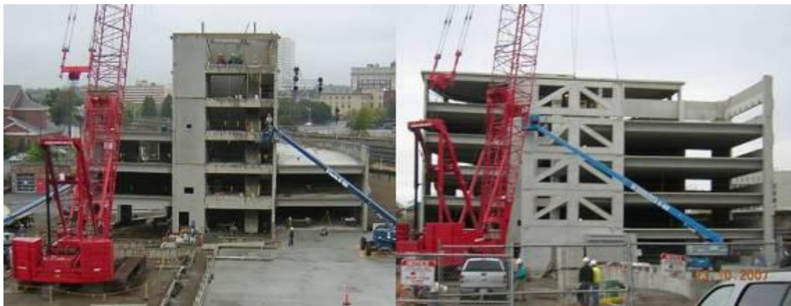
Figure 15 - Erection of Precast Structure: Oct. 10th, 2007 (left) & Oct 23rd, 2007 (right)
