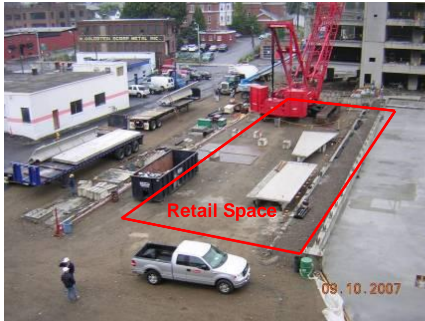
Figure 3 - Photo of construction site depicting retail space to be slabbed.
