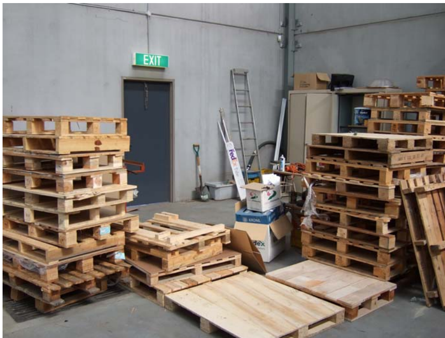
Figure -12-4: Obstructed Exit in Building F
