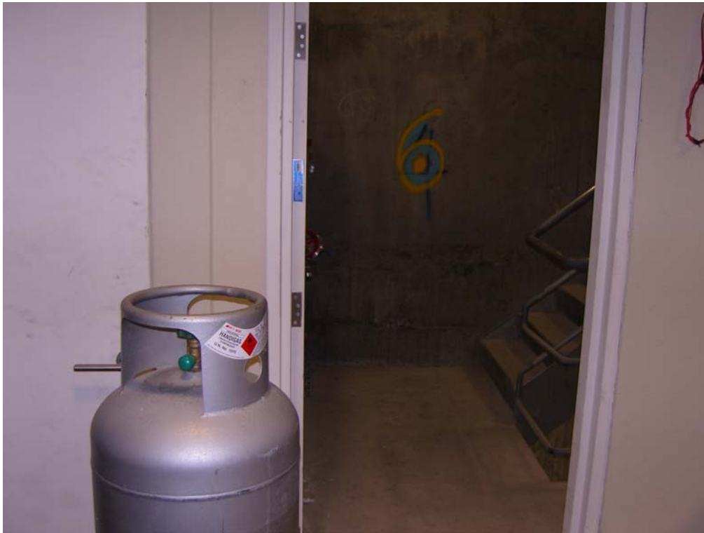
Figure 12-3: LPG Tank in Lift Lobby Outside Open Door to Stairway in Building C
