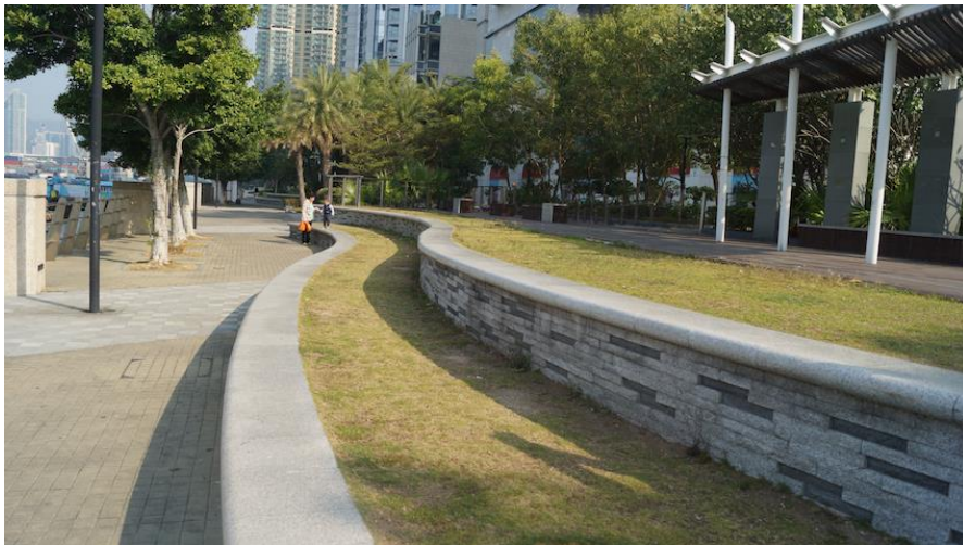
FIGURE 33: VIEW OF A SITTING AND PLAY AREA ALONG A TAI KOK TSUI PROMENADE. (COURTESY OF ALFRED SCOTT)
