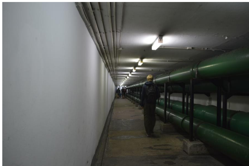
FIGURE 42: SUBWAY USED TO ACCESS NOONDAY GUN AREA. (COURTESY OF BETH LACARRA)
