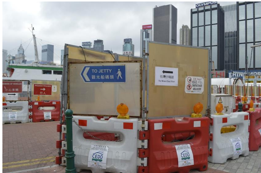
FIGURE 45: CONNECTIVE SIGNAGE AVAILABLE TO VISITORS TRAVELING BETWEEN WAN CHAI AND SURROUNDING AREAS. (COURTESY OF BETH LACARRA)
