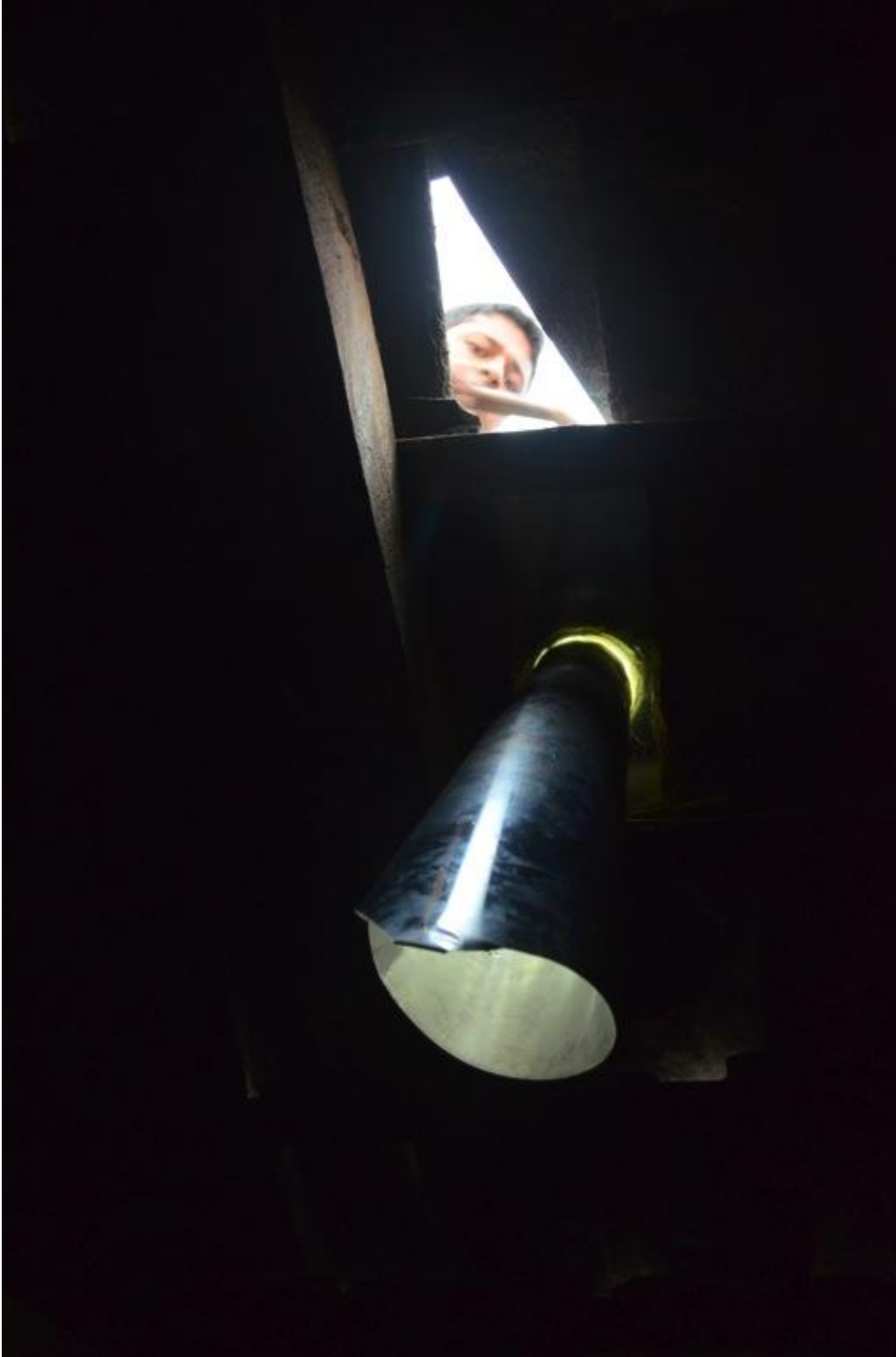
(An inside photo of the solar bottle cone base sheet being nailed into place on the roof)
