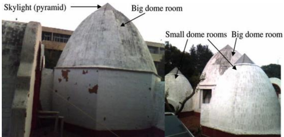
Figure 14: Dome rooms in IIT- Delhi (Chel et al, 2009)
