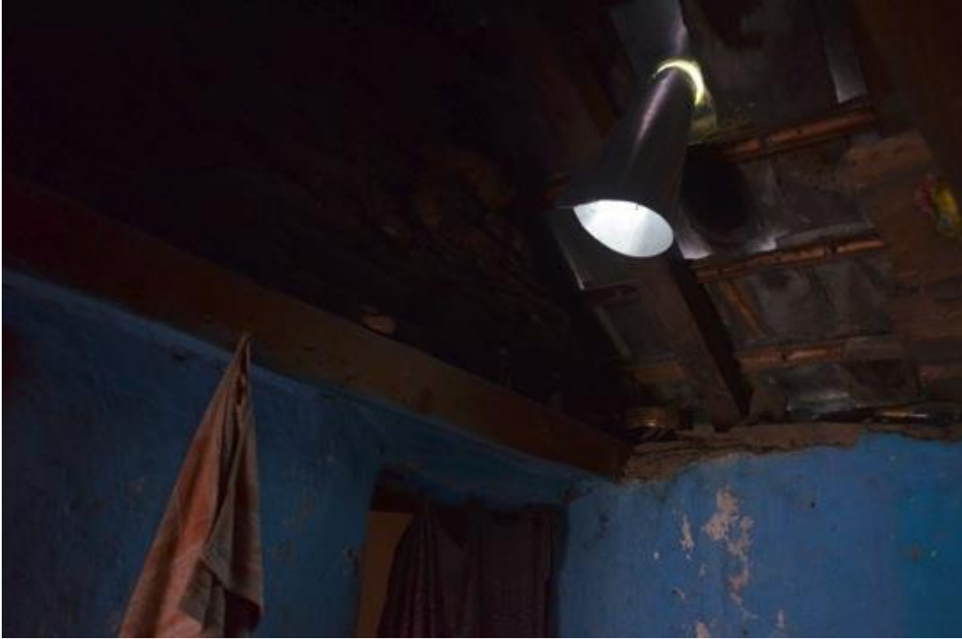
(Photo of the implemented solar bottle cone from inside the living room)
