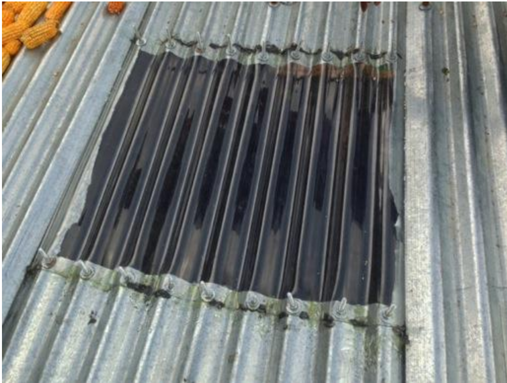
Figure 33: Photograph of the simple skylight prototype (Photo credit: Mert Can Erad, 2013)
