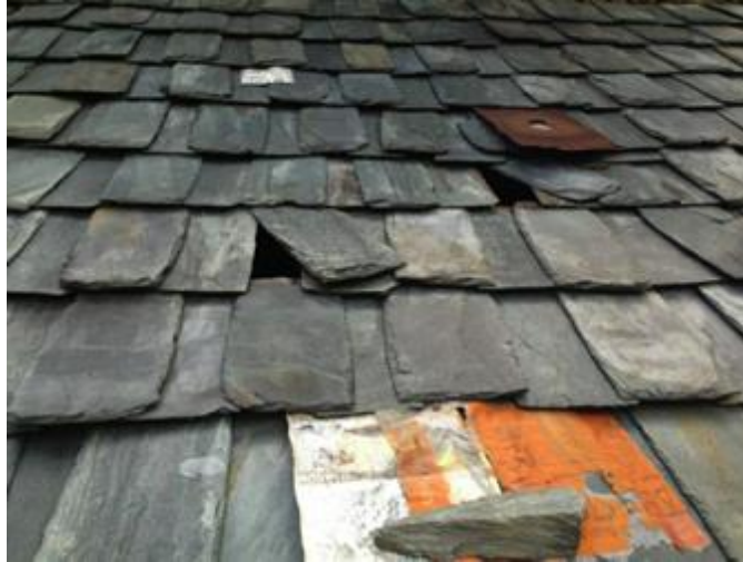
Figure 22: Terrace structure of the slate tiles (Photo credit: Mert Can Erad, 2013)
