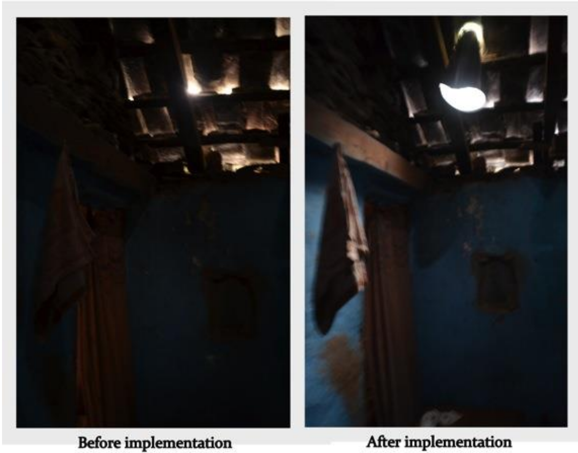
Figure 37: Fadle Village house #2 living room (Photo credit: Nehir Keskin, 2013)
