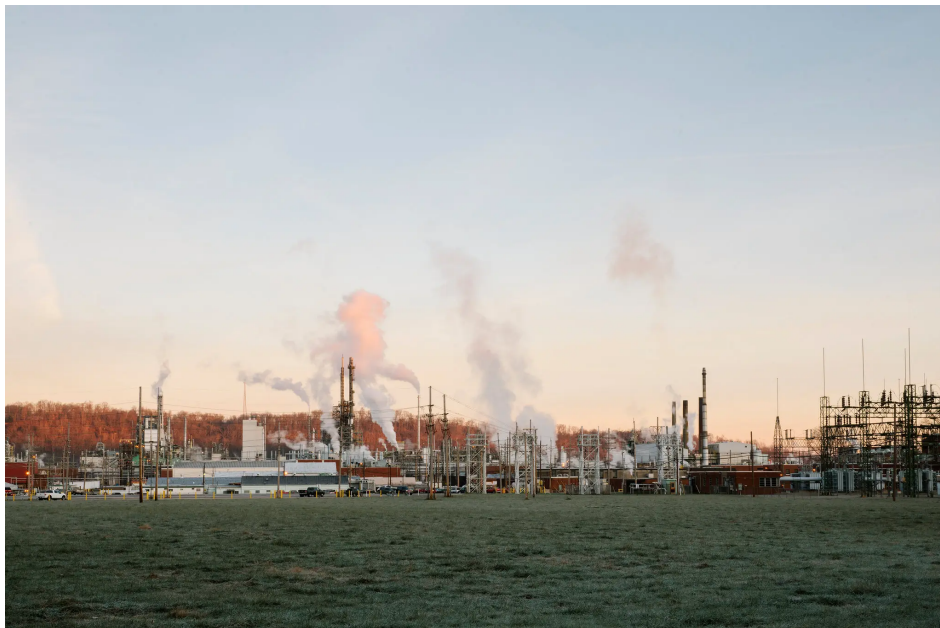
Figure 2. This is an image of the DuPont facility responsible for the disaster in Parkersburg, West Virginia (Rich, 2016).
