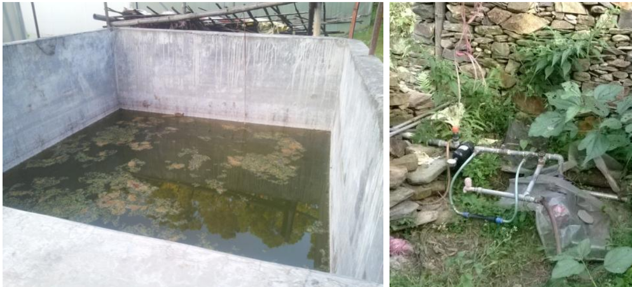
Figure 23: Water Tank Used for Poly-house (left), Water Travels through Pipes (right)
