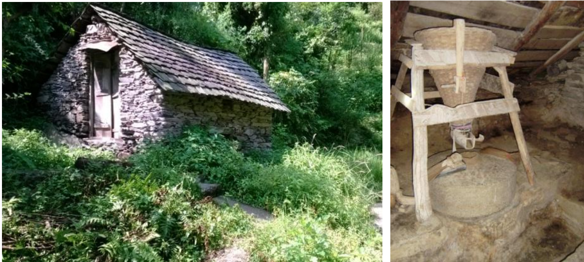
Figure 14: Stone-hut Mills in Kataula, Exterior (left), Interior (right)
