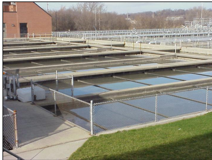
Figure 2.2: Simple Primary Wastewater Treatment (Settling Tank)
