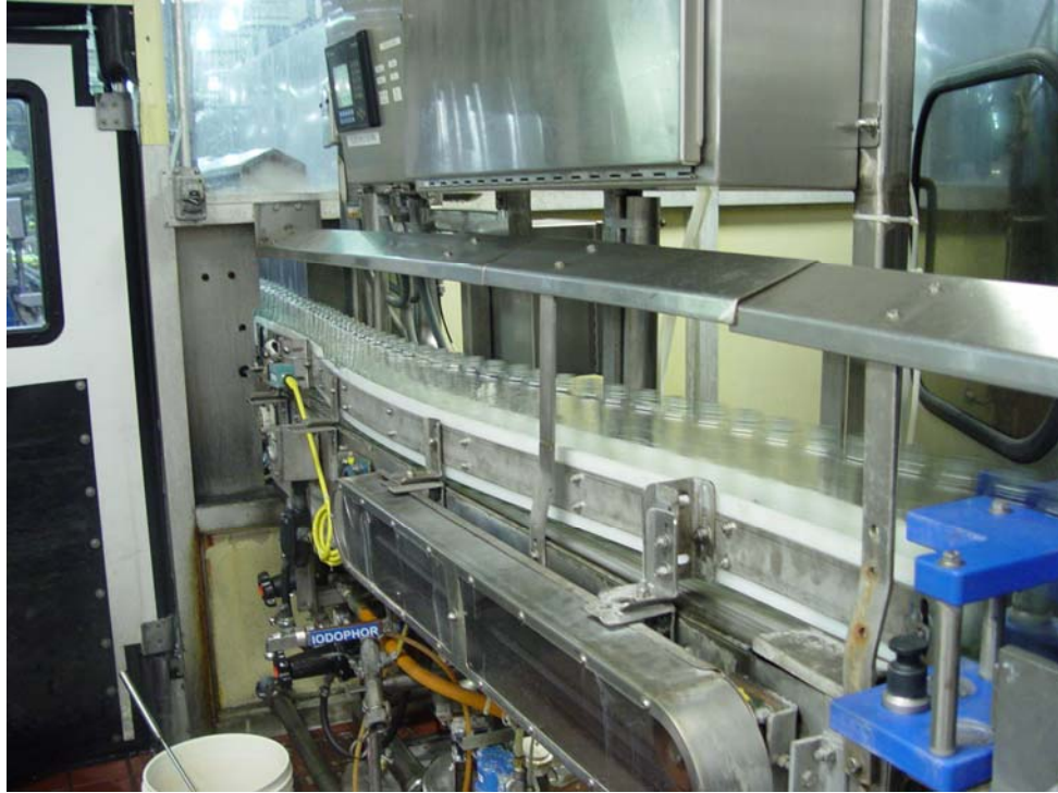
Figure 31 - Installation of New Pre-Filler Rails
