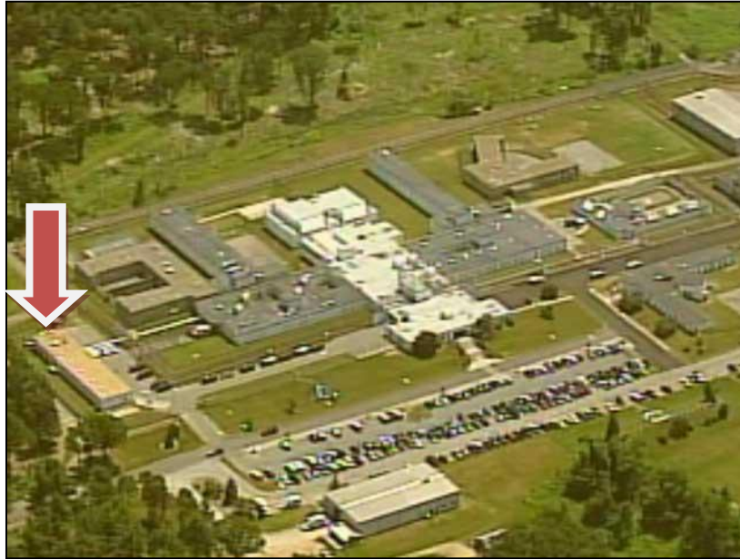
Figure 2.1 a: Worcester County Jail Site and Boiler Room Location (FOX25, 2012)
