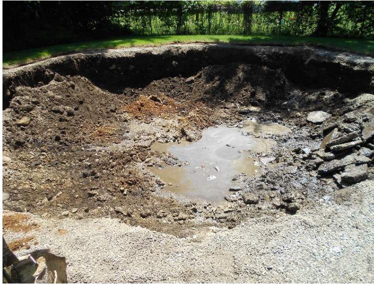
Figure 4: Removal of the Buckley's pool
