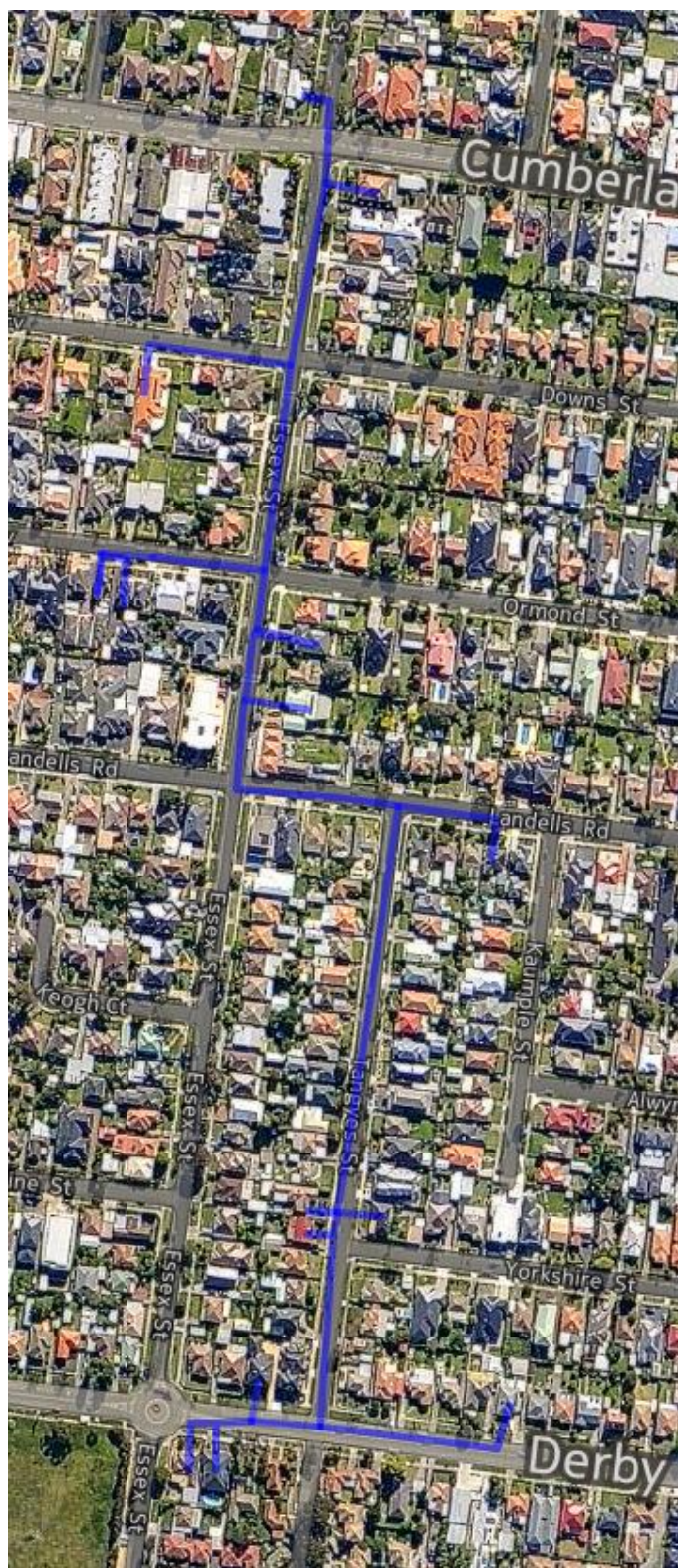
Figure 23. Nearmap image of Pascoe Value Homes with Solar Panels Installed
