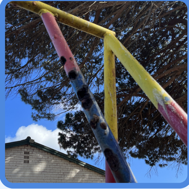
Holes in the swing set (top) and tunnel (bottom) from corrosion and unaffordable cost of maintenance
