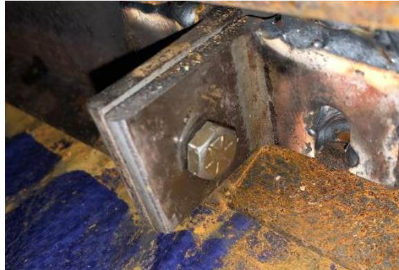
Figure 13: Angle iron with bolt and nut, used for joining modular frame sections.
