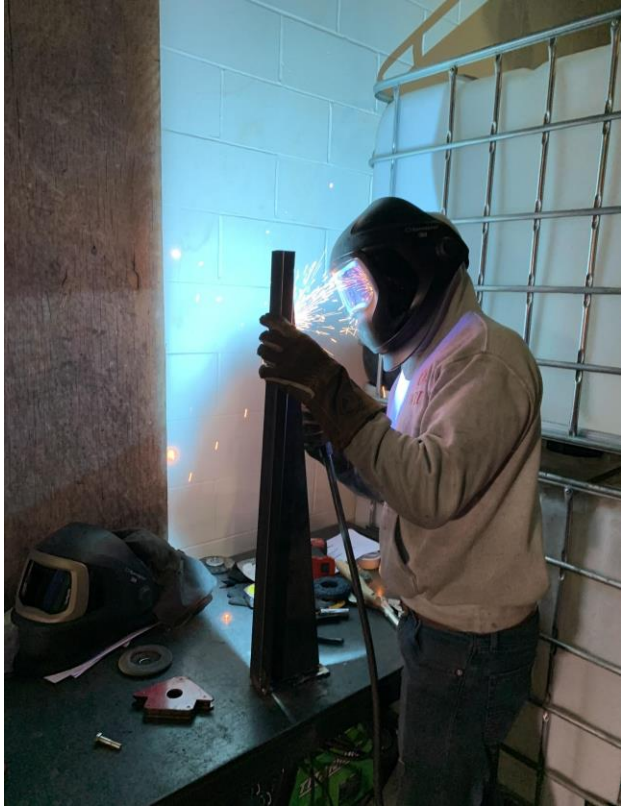
Figure 18: Buttruss being welded together
