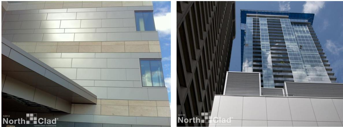
*Figure 1 - Examples of Rainscreens on Completed Structures [4]*
