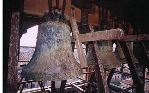
Figure 1 Bells covered in Pigeon droppings in Santa Fosca.
