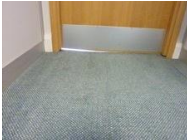
Figure 4: Rear fire escape door gap
