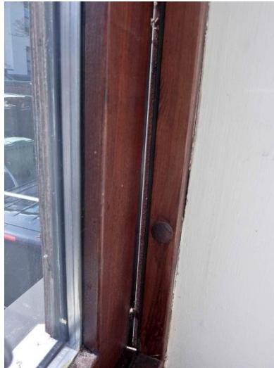
Figure 3: Warped window
