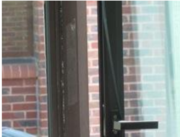
Figure 3: A window that had a seal falling off it. This is possibly an area for improvement.
