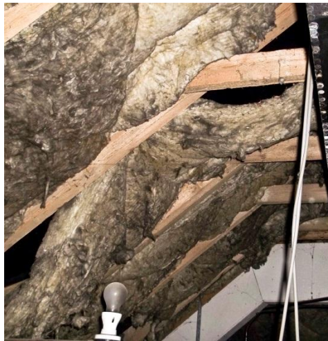
Figure 4: Insulation falling off the roof
