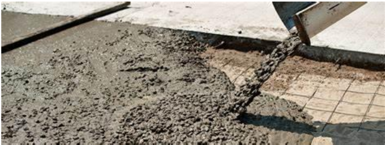
Figure 2: Wet Concrete (Omex, 2021)
