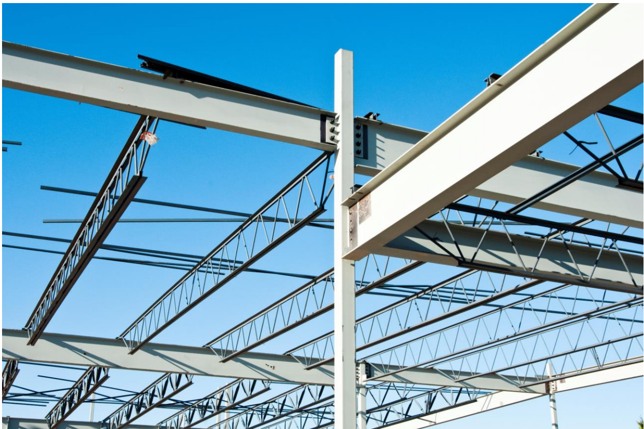
Figure 1: Steel Skeleton of a Building (Metinvest, 2022)
