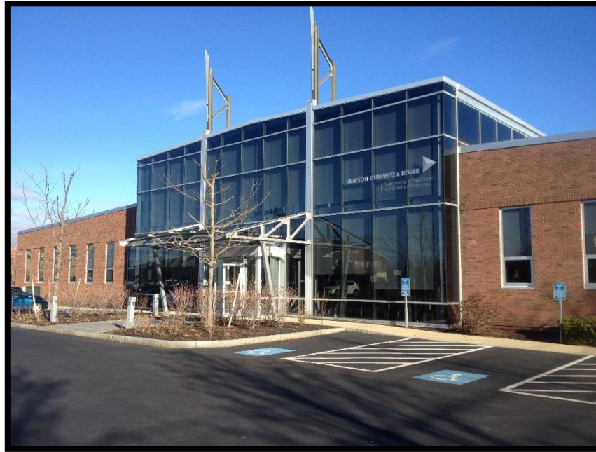
Figure 1.1: SGH Office, Waltham, MA
