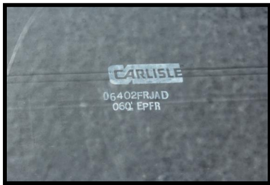
Figure 5.16: SGH Roof EPDM
