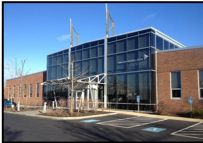
Figure 5.1: Southeast Façade of SGH Office Building
