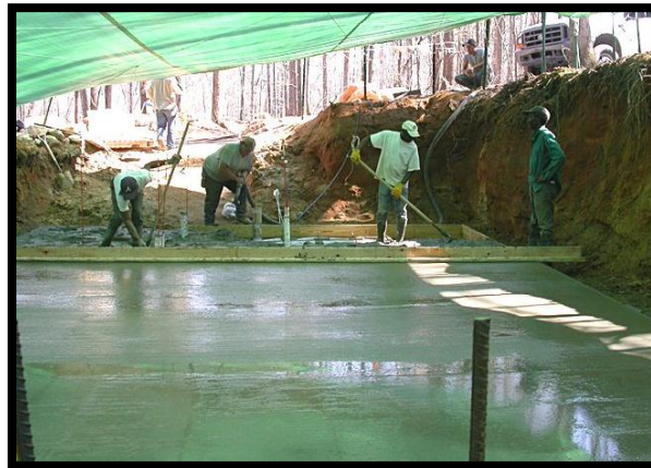
Figure 4: Pouring and Curing Concrete [15]
